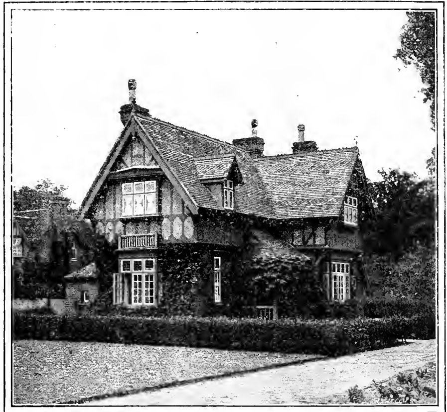
FIG. 59.—BAGSHOT PARK: THE GARDENER'S RESIDENCE.
