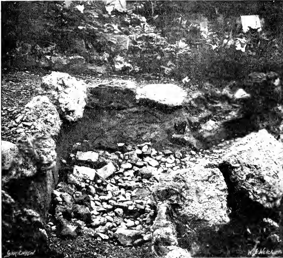
FIG. 52.—MORAINE GARDEN: SHOWING THE WATER-TIGHT WALLS AND MATERIALS FOR DRAINAGE.
