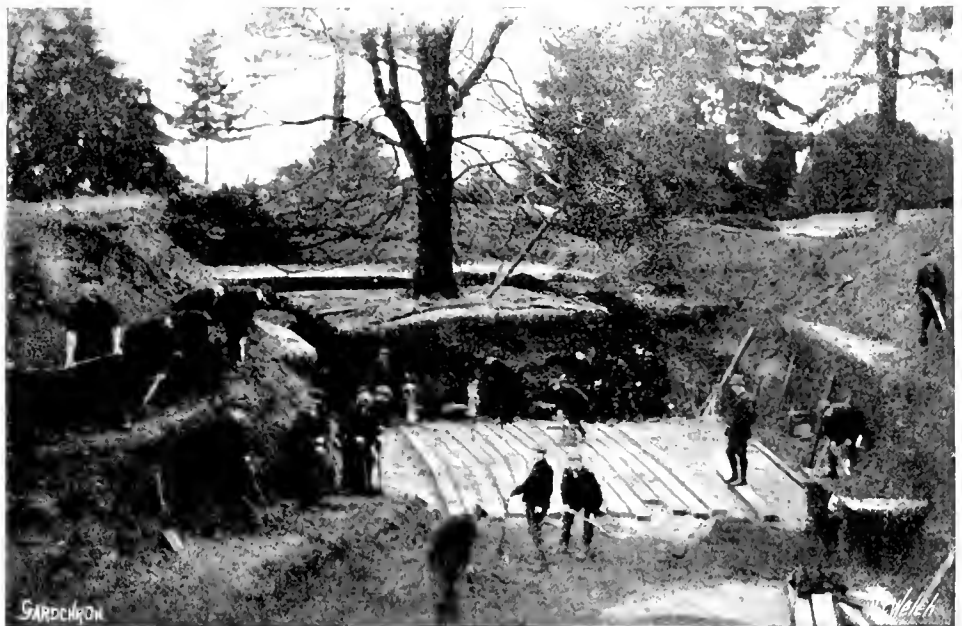
FIG. 64.—REMOVING A LARGE BEECH TREE AT WARREN HOUSE, MINLEY.
