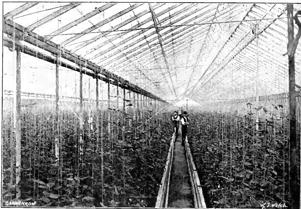
FIG. 80.—INTERIOR OF ROSE HOUSE AT THE DALE NURSERIES, CANADA.
