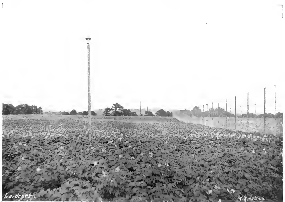
FIG. 107.—ELECTRIFIED AREA, DUMFRIES, 1913. LARCH POLES WITH INSULATORS SEEN IN THE CENTRE: THESE CARRY CHARGED OVERHEAD WIRES. ON RIGHT, WIRE NETTING ERECTED IN ORDER TO SCREEN THE CONTROL AREA.
