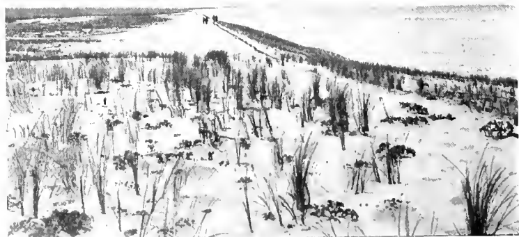
FIG. 123. ARTIFICIAL LITTORAL DUNE IN PROCESS OF FORMATION: PAVISAGE OF PLANKS JUST VISIBLE IN THE BACKGROUND.
