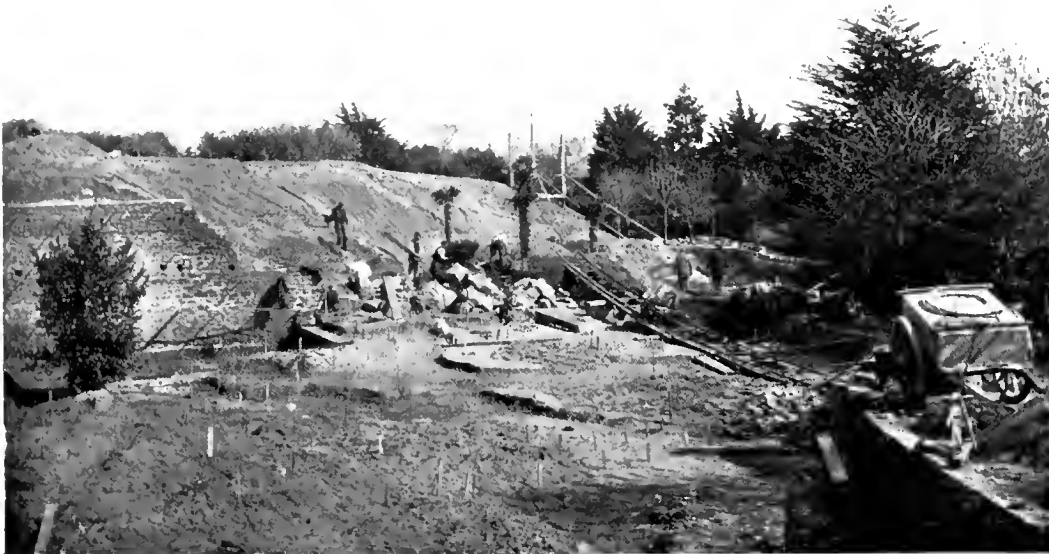
NO. 1.—A SUITABLE SITE FOR A ROCK GARDEN, SHOWING PREPARATORY WORK.
