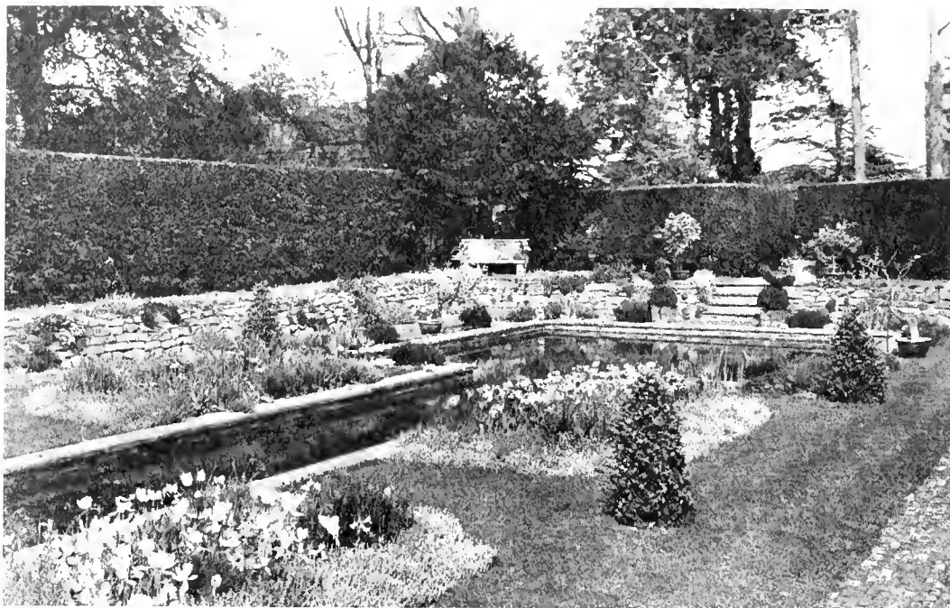
PART OF THE SUNK GARDEN AND LILY POND AT HALLINGBURY PLACE.
