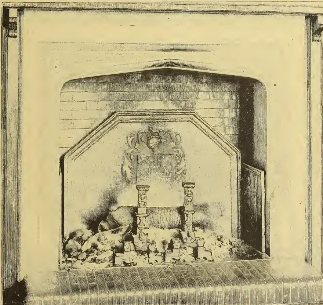
*Down fire for country house. In this the hearth of Ruabon brick is raised 10 inches above floor level. The fire-hearth is of cast iron. Fire-back, old Sussex. A simpler, bolder plan should be followed for working shed.*
