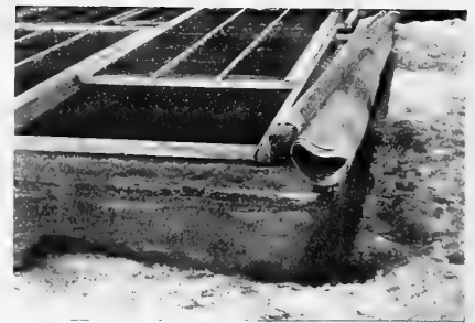
51. A roll of paraffined cotton cloth used to cover and protect the burlap mats
