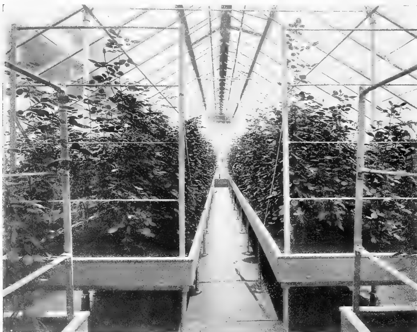
389. The best sort of greenhouse for the country gentleman. Larger than you want, perhaps, but built in the right way—for comfort, not for worry. The even-span house is the best for general purposes. The tall-growing American Beauty can be set in the centre benches. The heating pipes are under the benches, out of the way. The raised benches take less soil than solid beds, and are easily managed if carefully watered
