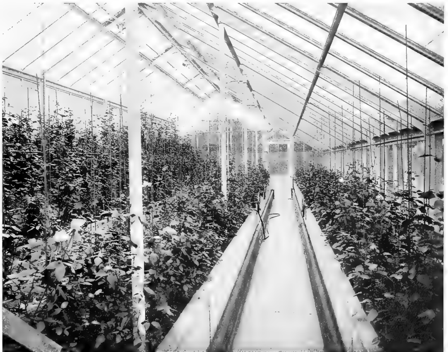
391. The three-quarter-span house is practical where a building wall can be made to do service. Solid beds are preferred to raised benches if the plants are to be carried over more than one season. A good example of modern construction—all iron and glass—permanent, free from drip, shadow and draughts, efficient, attractive and cheaper in the long run because a saver of coal and repair bills
