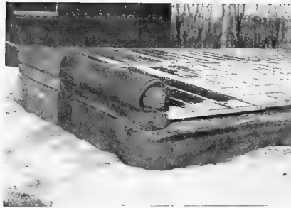
50. Threefold burlap mats instead of the old-style straw mats to keep out frost
