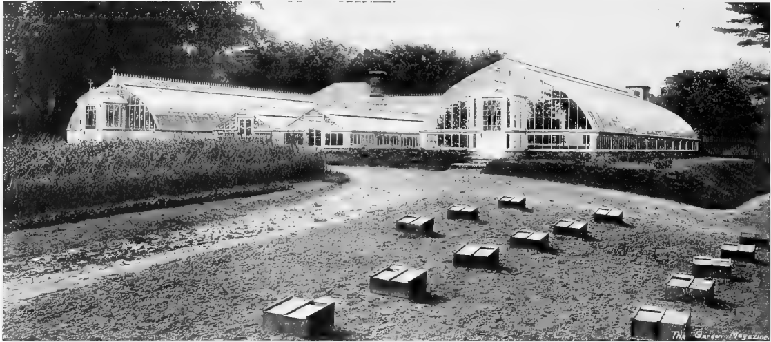
DESIGNED AND EXECUTED FOR T. C. EASTMAN, ESQ., TARRYTOWN, N. Y. SHOWING MELON FRAMES IN THE FOREGROUND.
