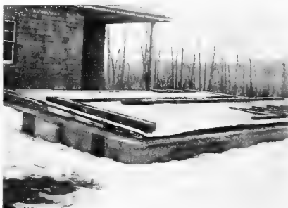
53. Covered for the night with the burlap mats and their paraffin cover
