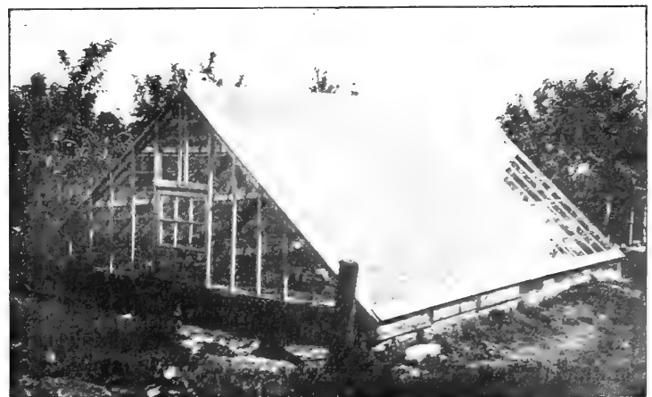
This little homemade greenhouse is heated by an inside slow combustion coal stove. Regulation sash bars are utilized for the roof
