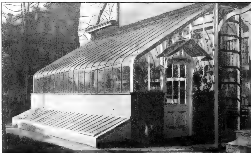
A lean-to greenhouse can be built in connection with the dwelling. Heated frames attached to this almost double the capacity
