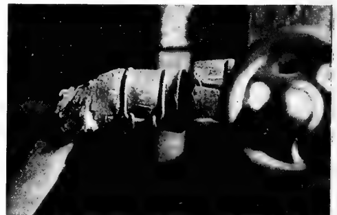
Pulling from the tap at a right angle is what wears out a hose
