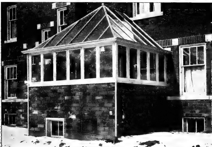
As the conservatory looks from the outside
