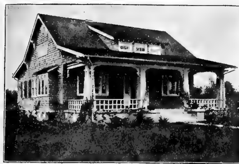
Stained with Cabot's Shingle Stains. Hollingsworth & Bragdon, Arch'ts, Cranford, N. J.
