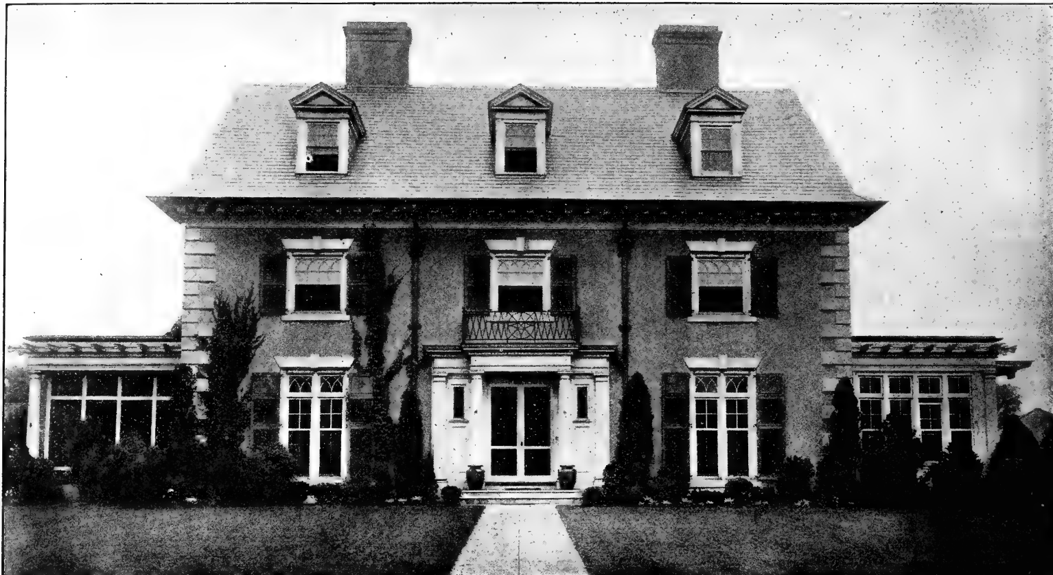
FOUNDATION PLANTING THAT IS TWELVE YEARS OLD
