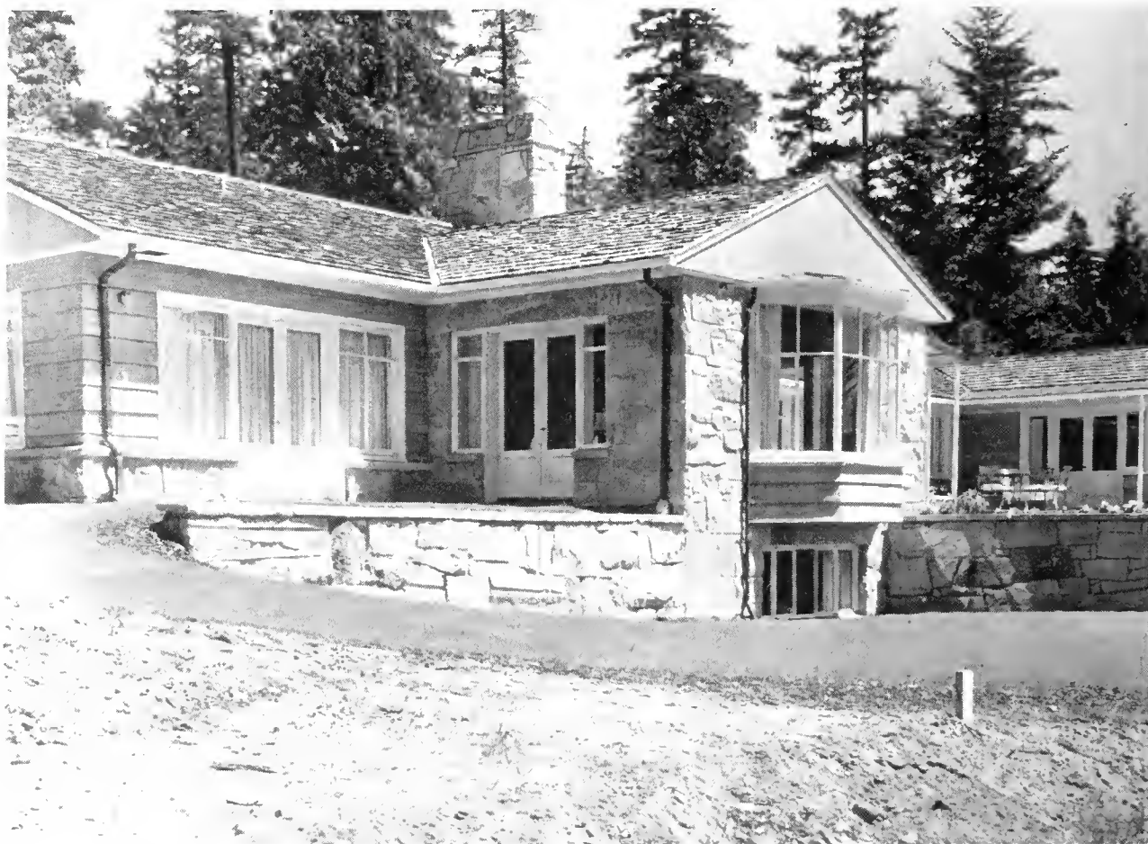
Immediately after construction of the Miller residence in 1949...
