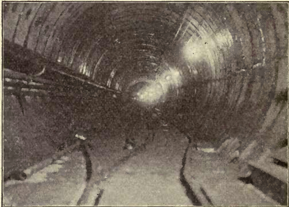
FIG. 367. — Interior of a Ten-foot Intake Water Tunnel.
