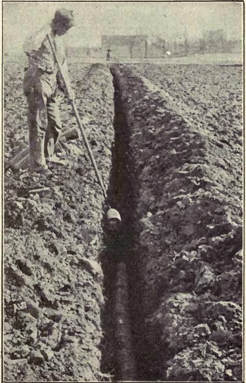
FIG. 267. — Tiling Level Lands, Illinois.
