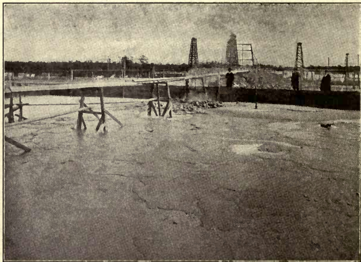
FIG. 224. — A Well Pumping Sulphur.
