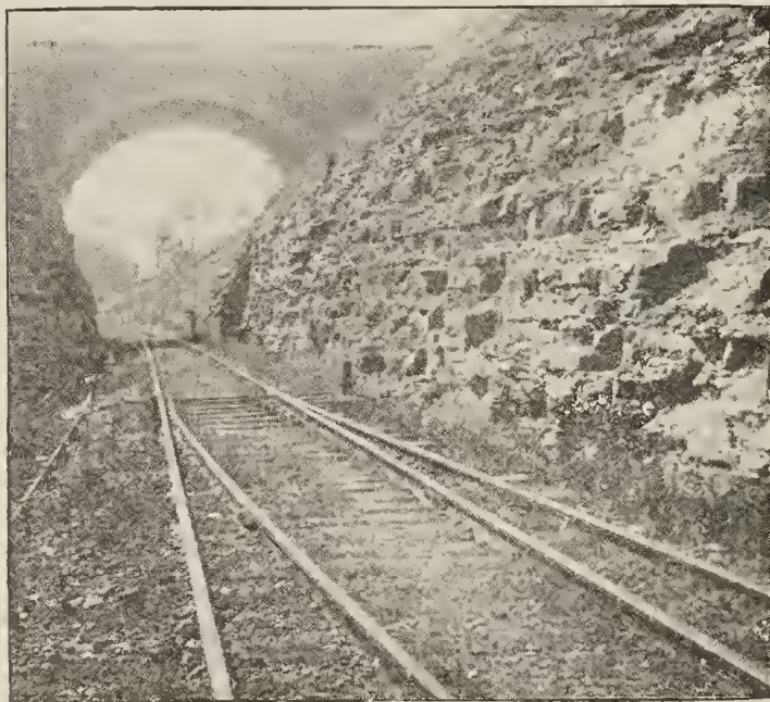
FIG. 36.—Stratified Triassic Beds exposed in a Railway Cutting, Gosford.
