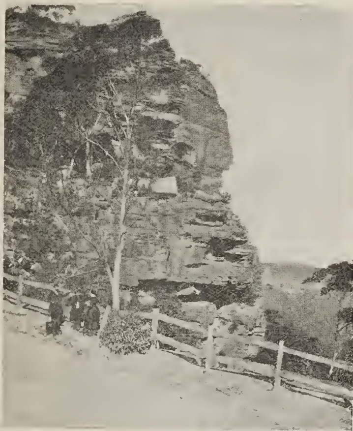
FIG. 18. —Mount Victoria Pass, Blue Mountains, showing how the stratified sandstones are cut under by Atmospheric agencies.
