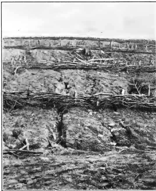
FIG. 77.— Rapid erosion of deforested land and one method of preventing further erosion. (U. S. Geol. Surv.)
