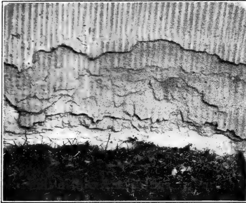
FIG. 3. — Sandstone "set on edge," showing the scaling of the laminae by frost.
