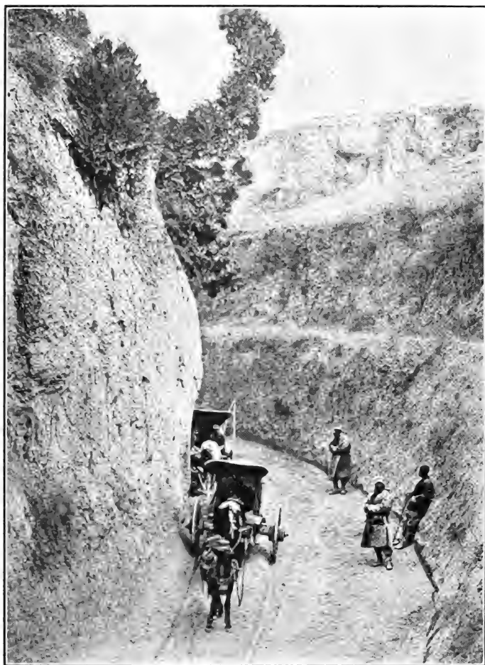
FIG. 31. — Loess deposits, Shan-si, China. The canyon-like depression was excavated by the wind as the loess was loosened by traffic. The two levels on the right are old roads. The ability of loess to stand in almost vertical walls is shown. (Carnegie Institution.)
