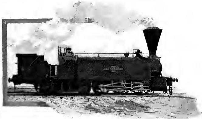
Abb. 266. Locomotive System Engerth. [Cockerill 1853.]
