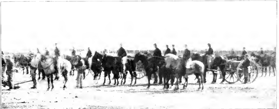
READY TO OPEN FIRE IN THE TRENCHES
