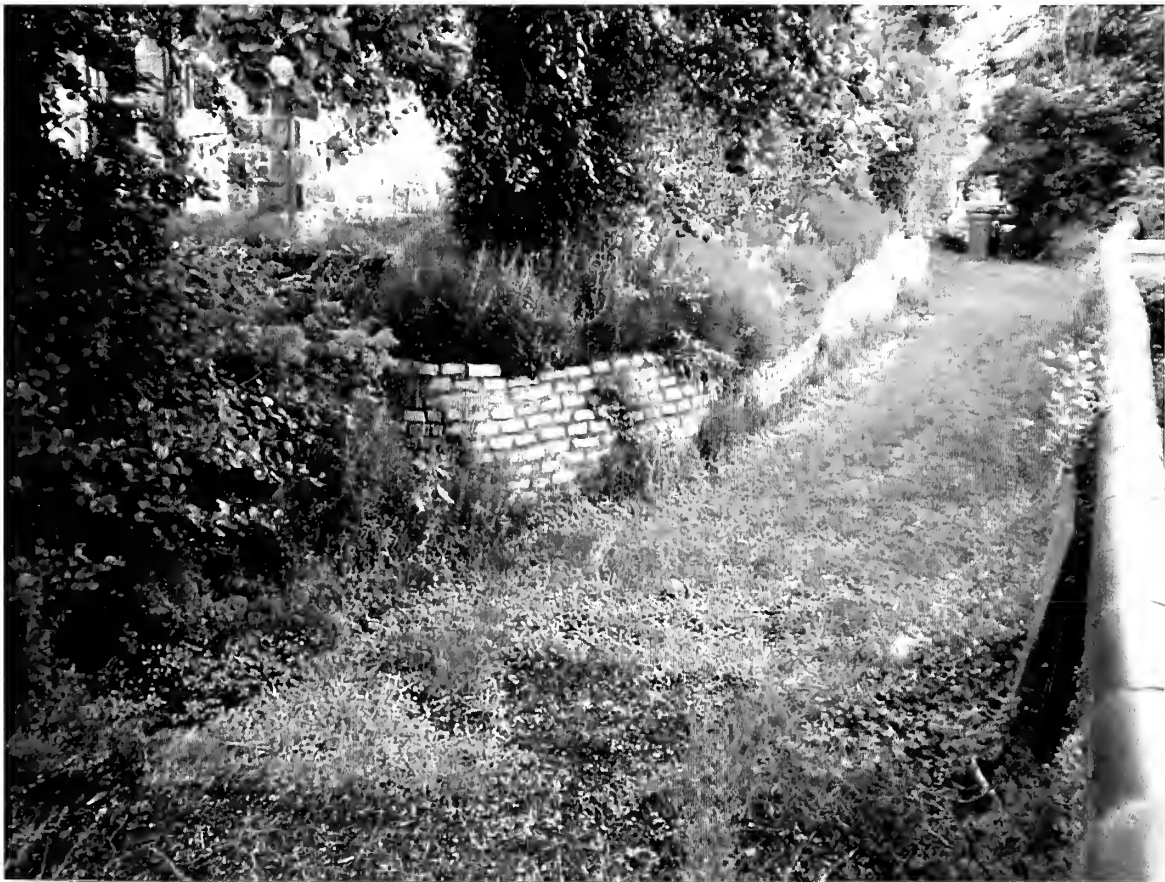
Fig.2. Newark Drive - Grassed over concrete driveway.
