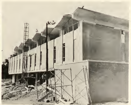
add a little cement and brick on the outside . . .
