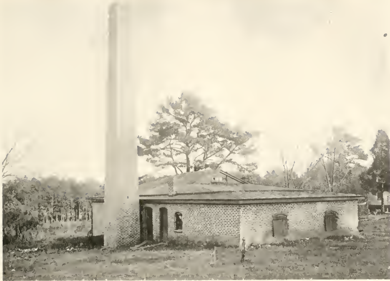
Old Heating Plant
