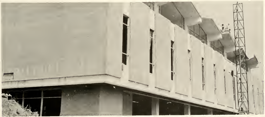
The Union Building Under Construction
