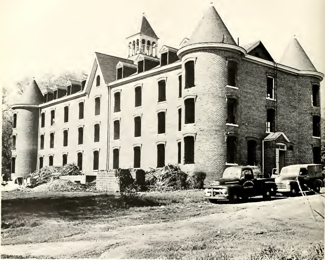
Carter Hall under re-construction
