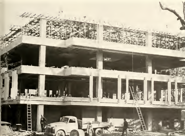
Men's dormitory now under construction
