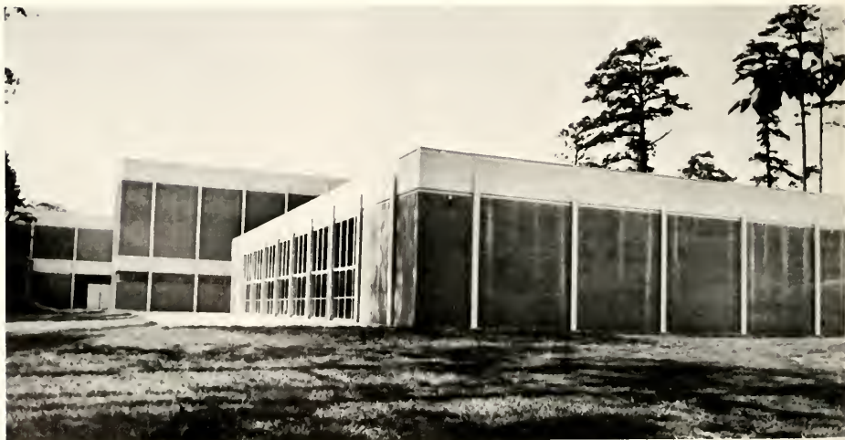
The new Hartley Woods Gymnasium.
