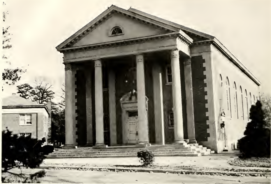
The Jane M. Smith Memorial Church, located near the entrance to the campus, is a gift of the late Mrs. Jane Berry Smith. This structure, built of colonial brick with limestone trimming, has a front supported by limestone columns. The structure is one of the most beautiful of its kind to be found on the campus of any college in America.
