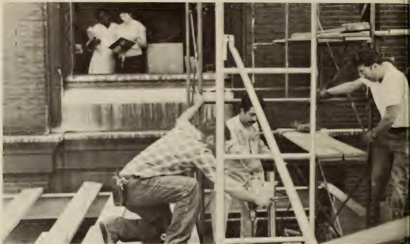
Working on the bridge connecting the Library and the Photo Collection are, left to right, Carl Hilgers, Fernando Rivera, and Al Sigler of the Museum's Department of
