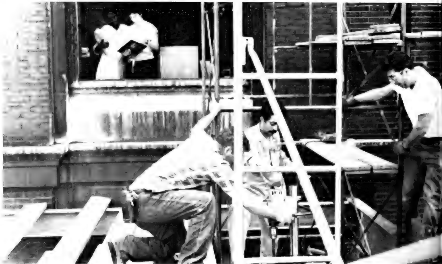
Working on the bridge connecting the Library and the Photo Collection are, left to right Carl Hilgers, Fernando Rivera, and Al Sigler of the Museum's Department of
