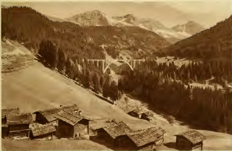
Langwies Viaduct (Coire-Arosa-Railway) the largest ferro-concrete bridge in the world. 313,7 yards long, principal arch 109 yards span.
