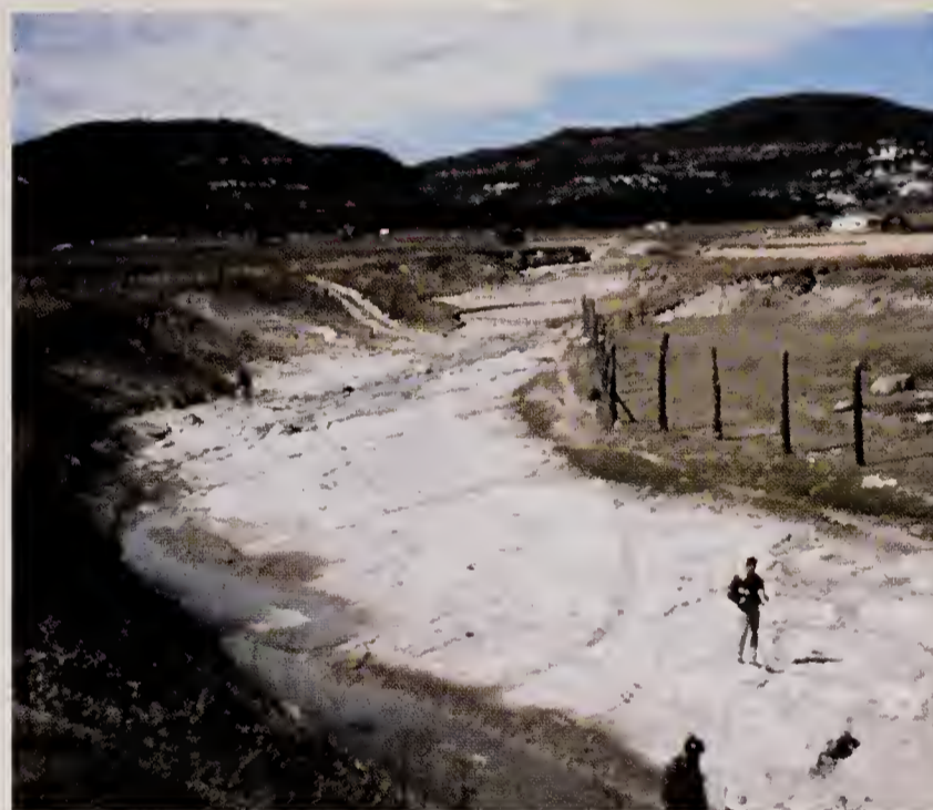
Figure 2. Bank erosion caused by a bedrock channel bottom. (Photo by J. Staats, NRST.)
