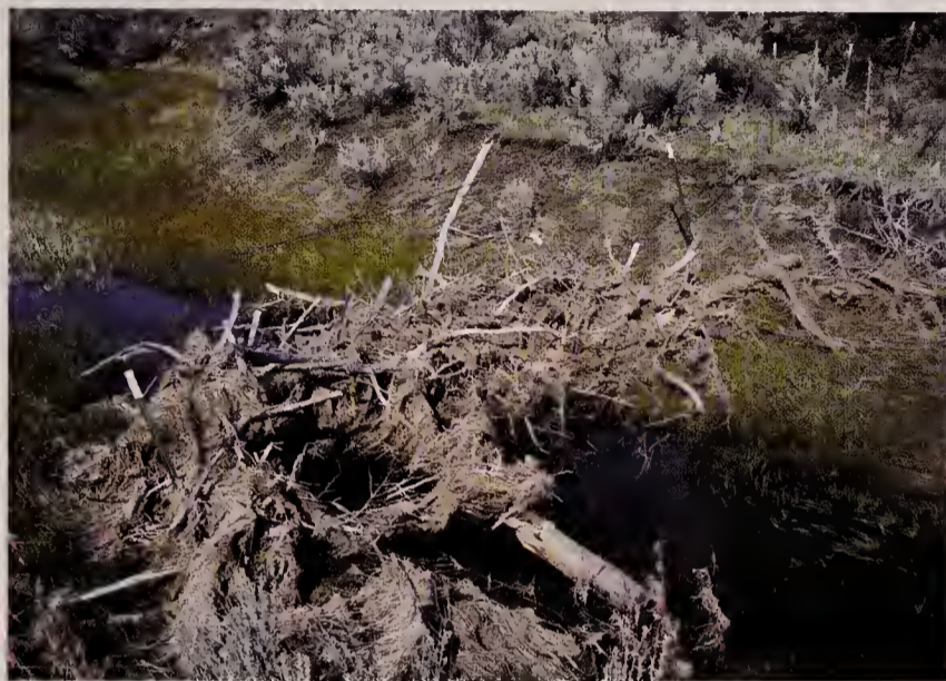
Figure 19. Cross fence collecting debris is susceptible to washing out. (Photo by S. Wyman, NRST.)
