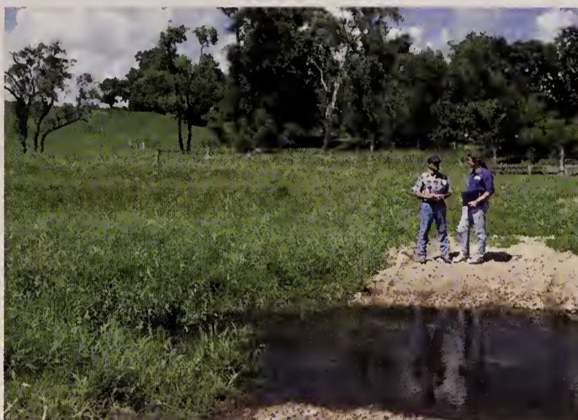
Figure 27. Hardened livestock crossing on a class 1 trout stream in Columbia County, Wisconsin (2000). (Photo by B. Nichols, NRCS.)
