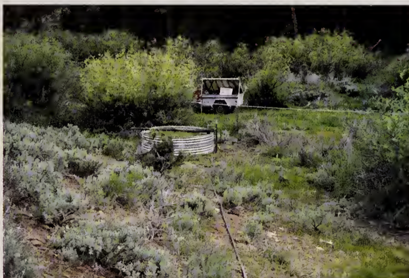
Figure 21. Mobile solar powered pump and tank. (Solar pump photos by D. Chamberlain, OSU Extension.)
