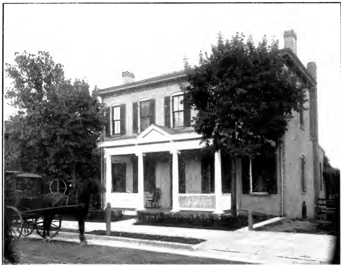
RESIDENCE OF J. C. GAUCH, President of Gundlach and Company, High and A Streets, 616 South Fourth Street.
