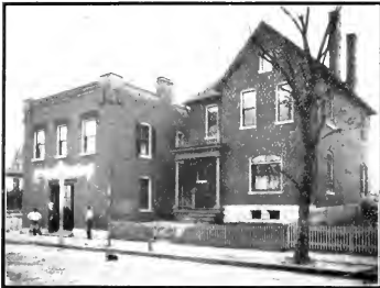
RESIDENCE OF JOHN KREHER, North High Street.
