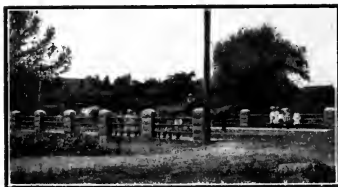
NEW BRIDGE AT CENTREVILLE AVENUE.
