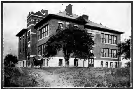
THE NEW RAAB SCHOOL BUILDING.
