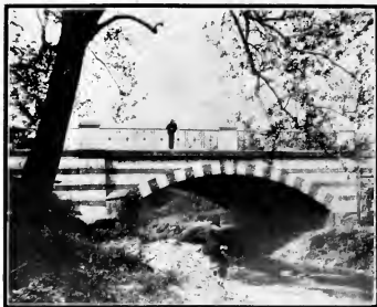
BRIDGE OVER THE RICHLAND CREEK.
