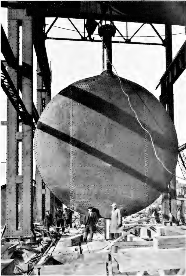
Niagara Falls. Butterfly valve to control water flow. Courtesy of the Niagara Falls Power Company
