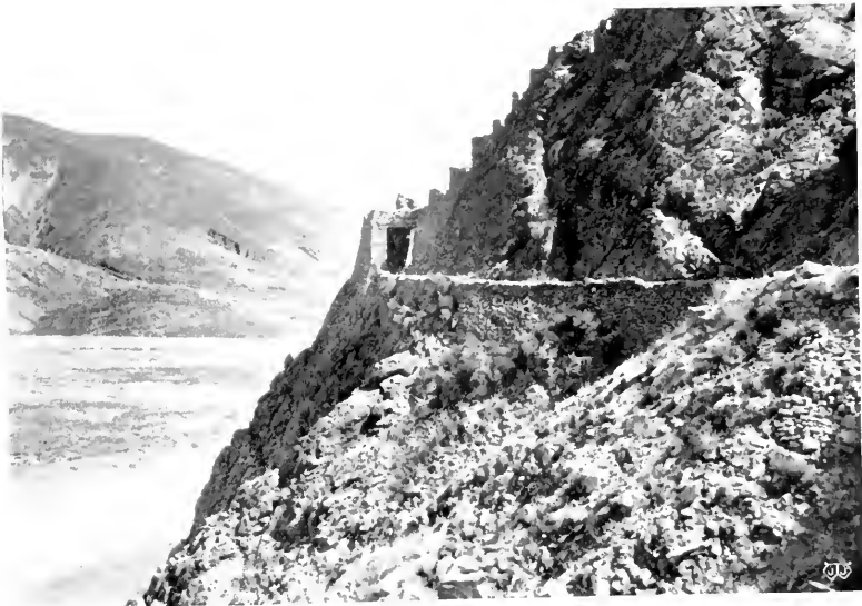
FORTIFIED WALL ACROSS THE ROAD NEAR PIN-DZO-LING.
