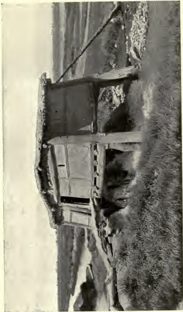
A PICTURESQUE FLOUR MILL AT SHWEIMO KWAN, KANSU. Many of these horizontal wheel constructions are seen in North-West China.
