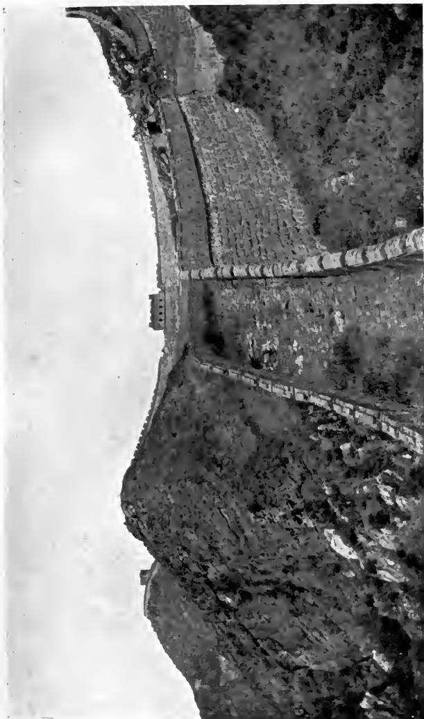
NORTH-EAST OF THE "THIRTEEN TOMBS," SHOWING DOUBLE PARAPETS FOR REVERSIBLE DEFENCE.
