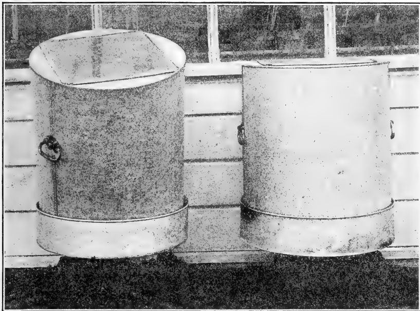
FIG. 1.—Glass-topped galvanized-iron moist chamber used for seedling plants.
