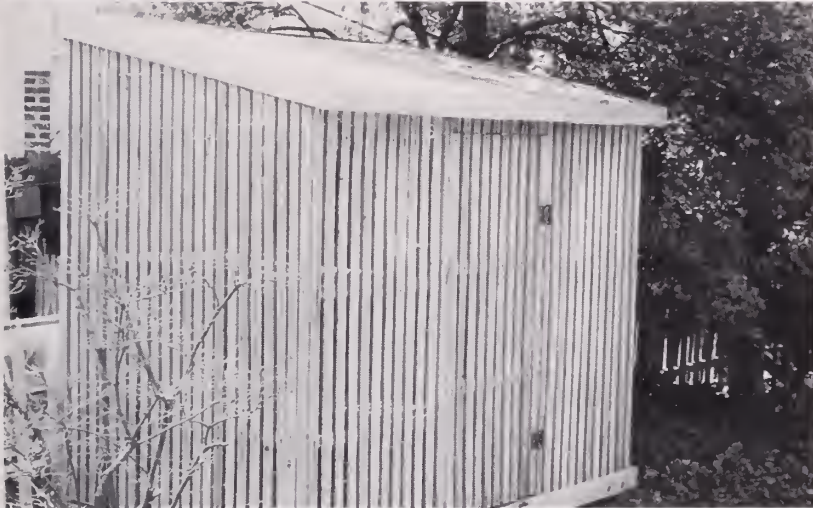
The Shutt's lath house, which is in scale with their small garden, can be locked.
