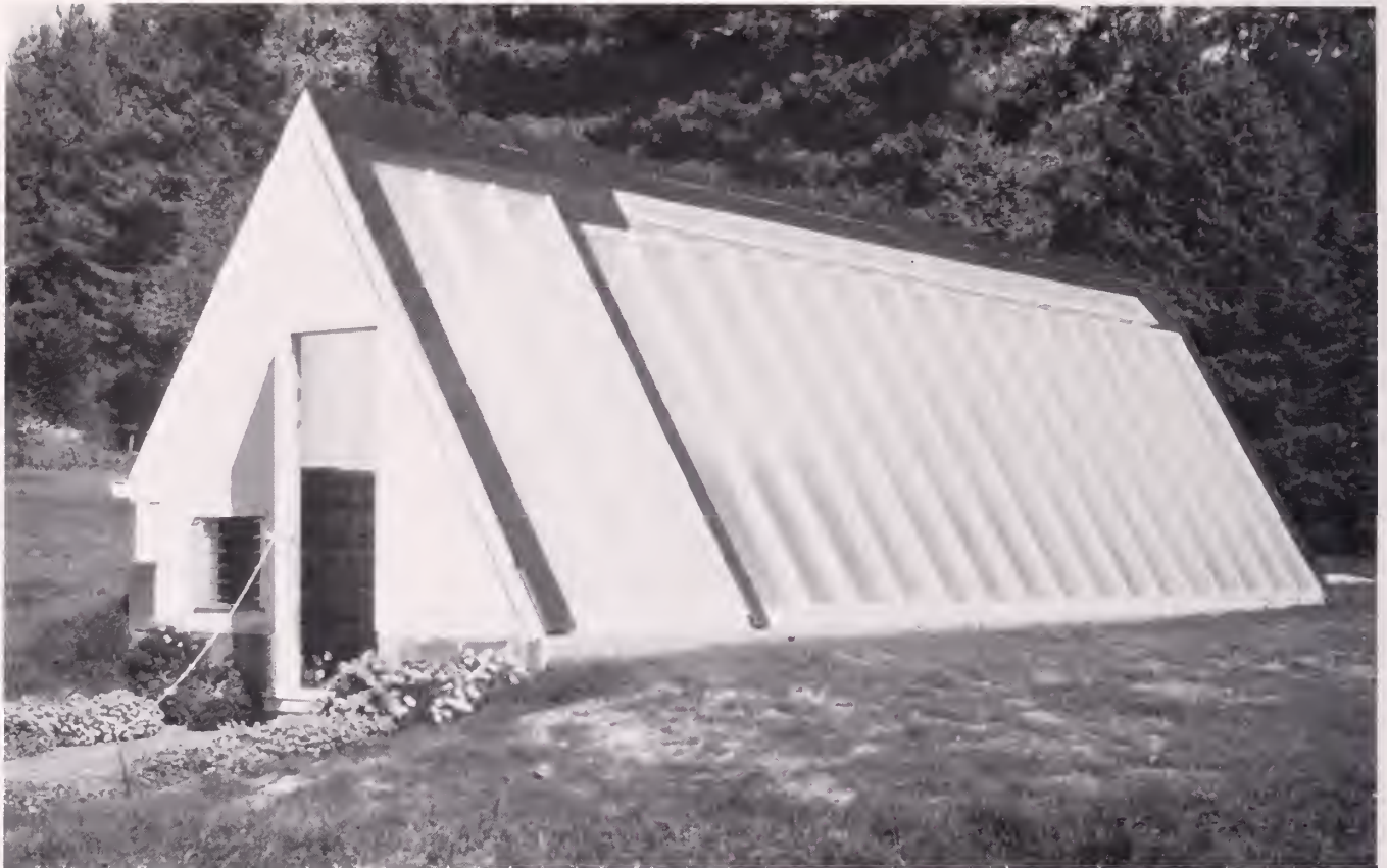
Passive solar pit greenhouse
