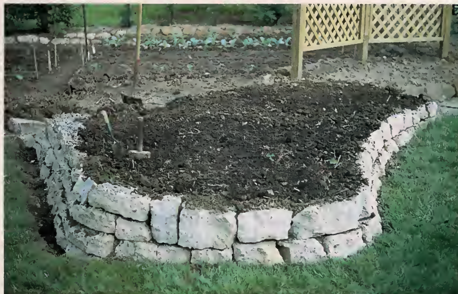
The brokrete of the raised bed is in place.
