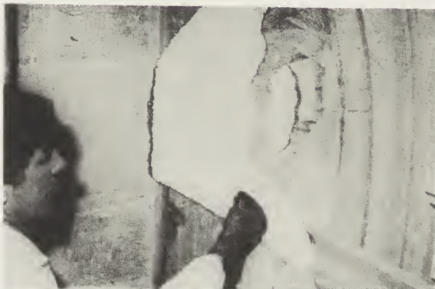
18) application of cellulose-paste with ammonium carbonate.
