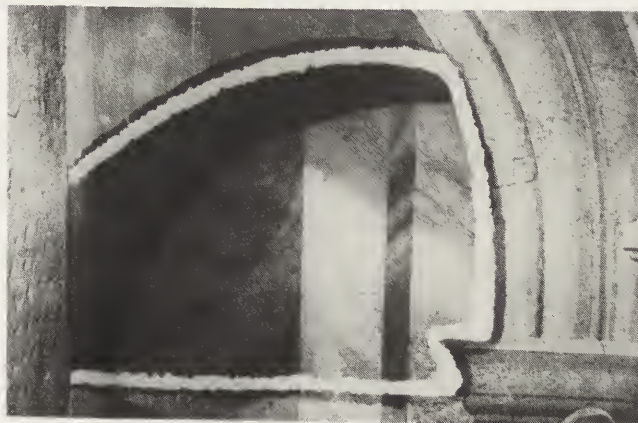
19) after the cleaning.
