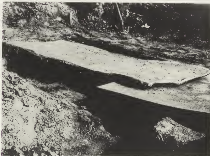
Figure 1 Separating the temporarily stabilized mosaic surface from the terrazzo embedment
