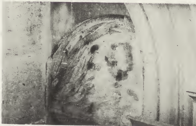
17) during the application of ammonium carbonate, applied with brush.
