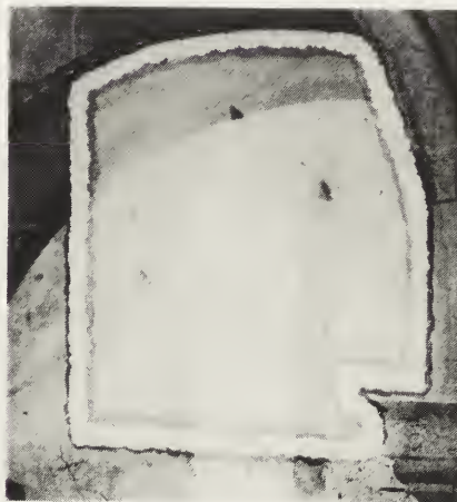
20) preparation for the consolidation with barium hydroxide.
