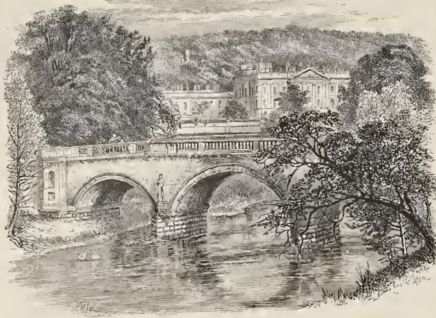
CHATSWORTH: WEST FRONT AND BRIDGE.
