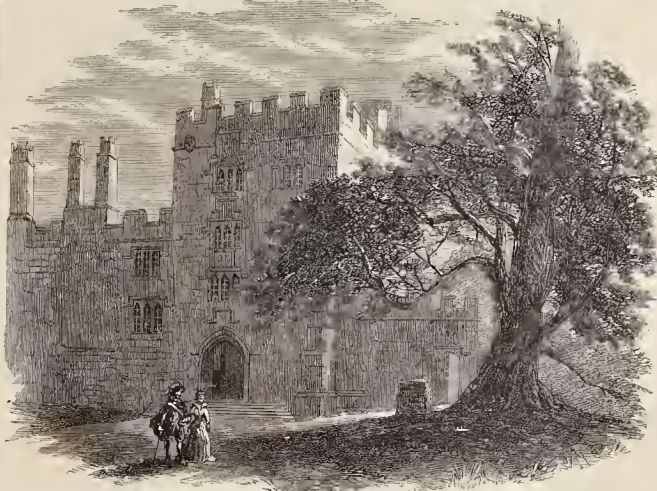
HADDON: THE MAIN ENTRANCE.
