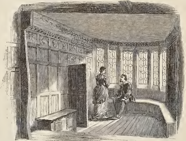
THE GRIEL WINDOW DINING-ROOM.
