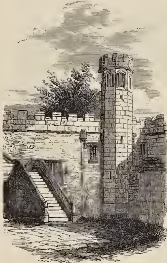
STEPS TO SIATE APARTMENTS.
