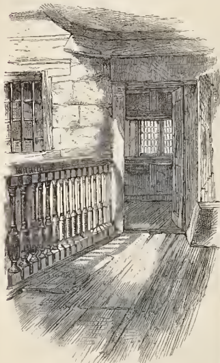
GALLERY ACROSS SMALL YARD.
