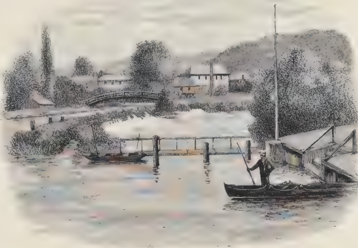
No. 21.—Marlow Weir.
