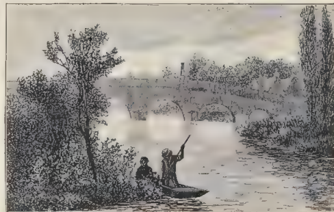
No. 28.—Chertsey Bridge.
