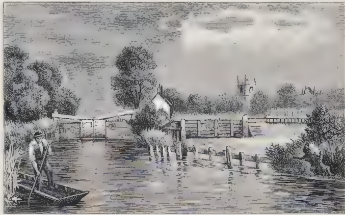
No. 11.—Benson Lock and Weir.
