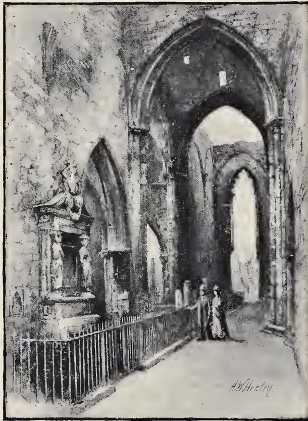
Transept, looking South.
