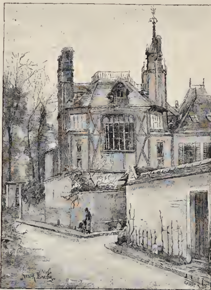
Another View of the Château.
