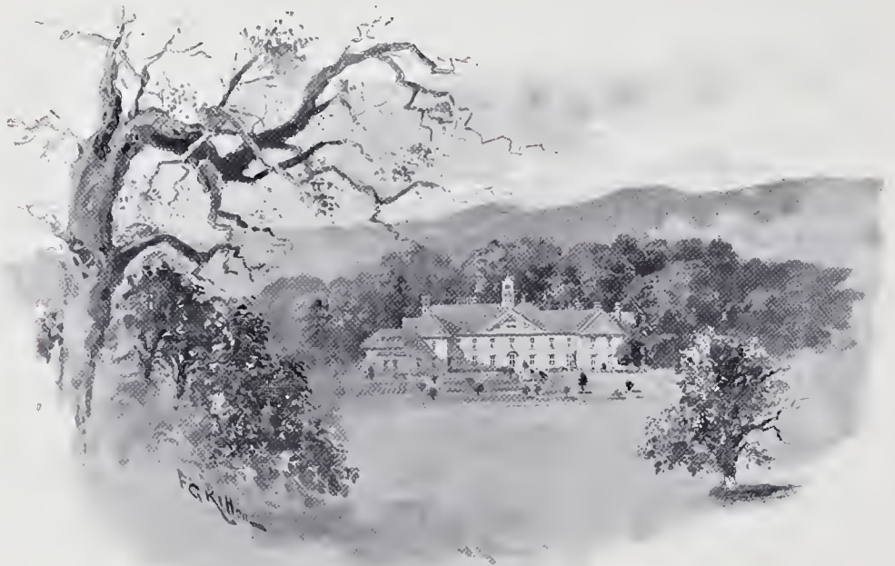
The Priory, Reigate.
