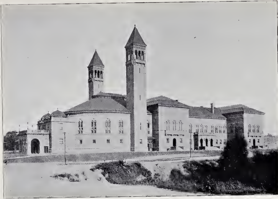
The Carnegie Art Gallery, Pittsburgh, Pennsylvania. Messrs. Longfellow, Alden and Harlow, Architects.
