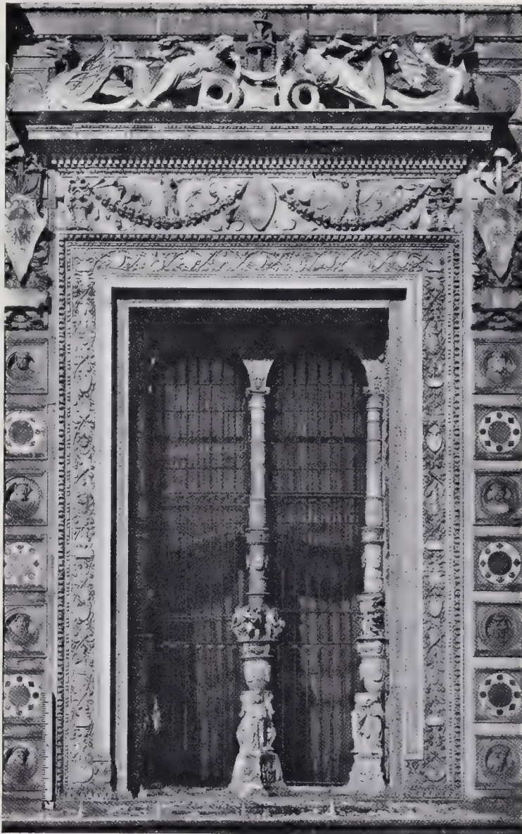
Window in the Façade.
