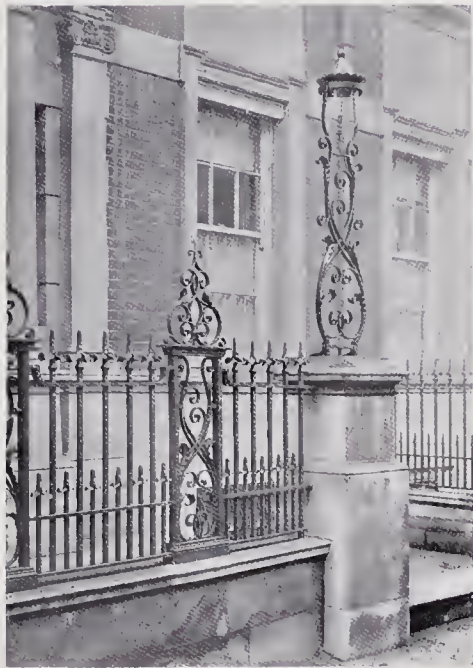
Forged Iron Railing and Standard at 32, Green Street, Park Lane for the Rt. Hon. Lord Ribblesdale.
