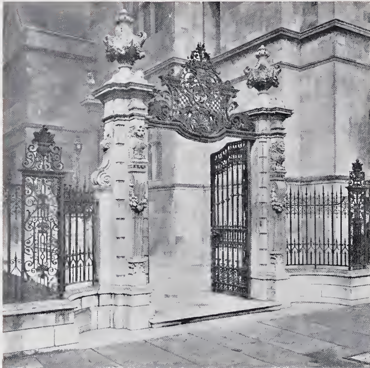
Gates, Railings and Grille at the Astor Estate Office, Victoria Embankment, for W. Waldorf Astor, Esq.
