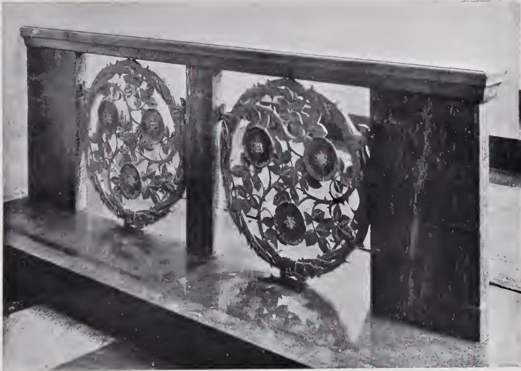
Altar Rail: subject, the Glorified Crown or Thorns. Rail, oxidised grey copper panels in brass uprights, dark Irish green marble; step, dark grey fossil marble.
