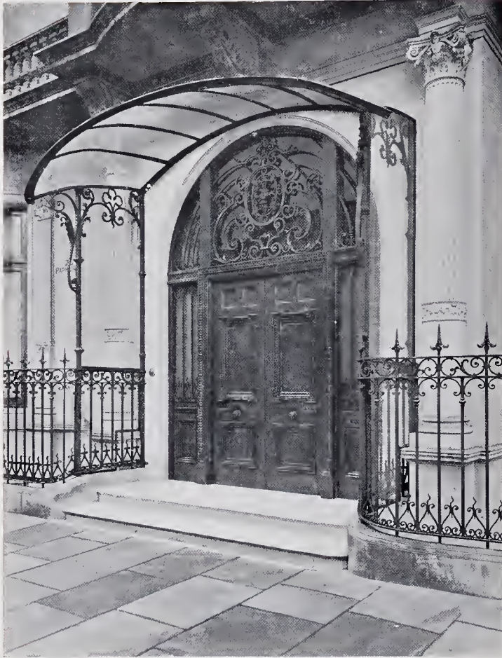
Porch at 25, Park Lane for Sir Edward A. Sassoon, Bart.
