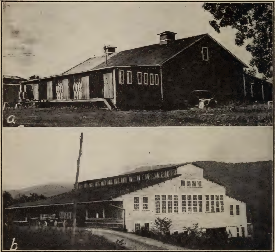
FIG. 15. (a) A western New York community packing house. The fruit is received at the left, packed through the house, and loaded on a railroad siding at the right. Two doors for unloading or for removing culls are available around the left corner. The lighting arrangement for packing is very poor. (b) This is a Maryland packing house. The packed fruit goes onto cars at a lower level on the right. The lighting is excellent.
