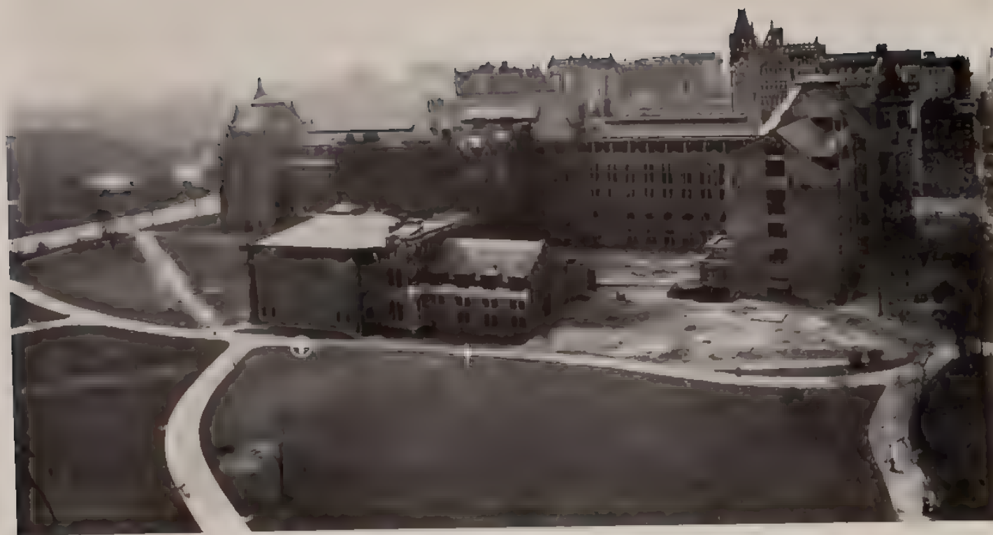
THE MUSEUM—REAR VIEW OF BUILDING. † Heating and Lighting Plant. ⊕ Lecture Hall
