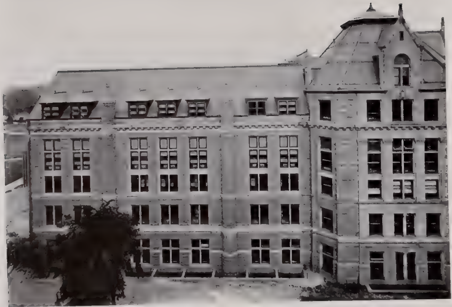
THE MUSEUM. South Wing of West Façade
