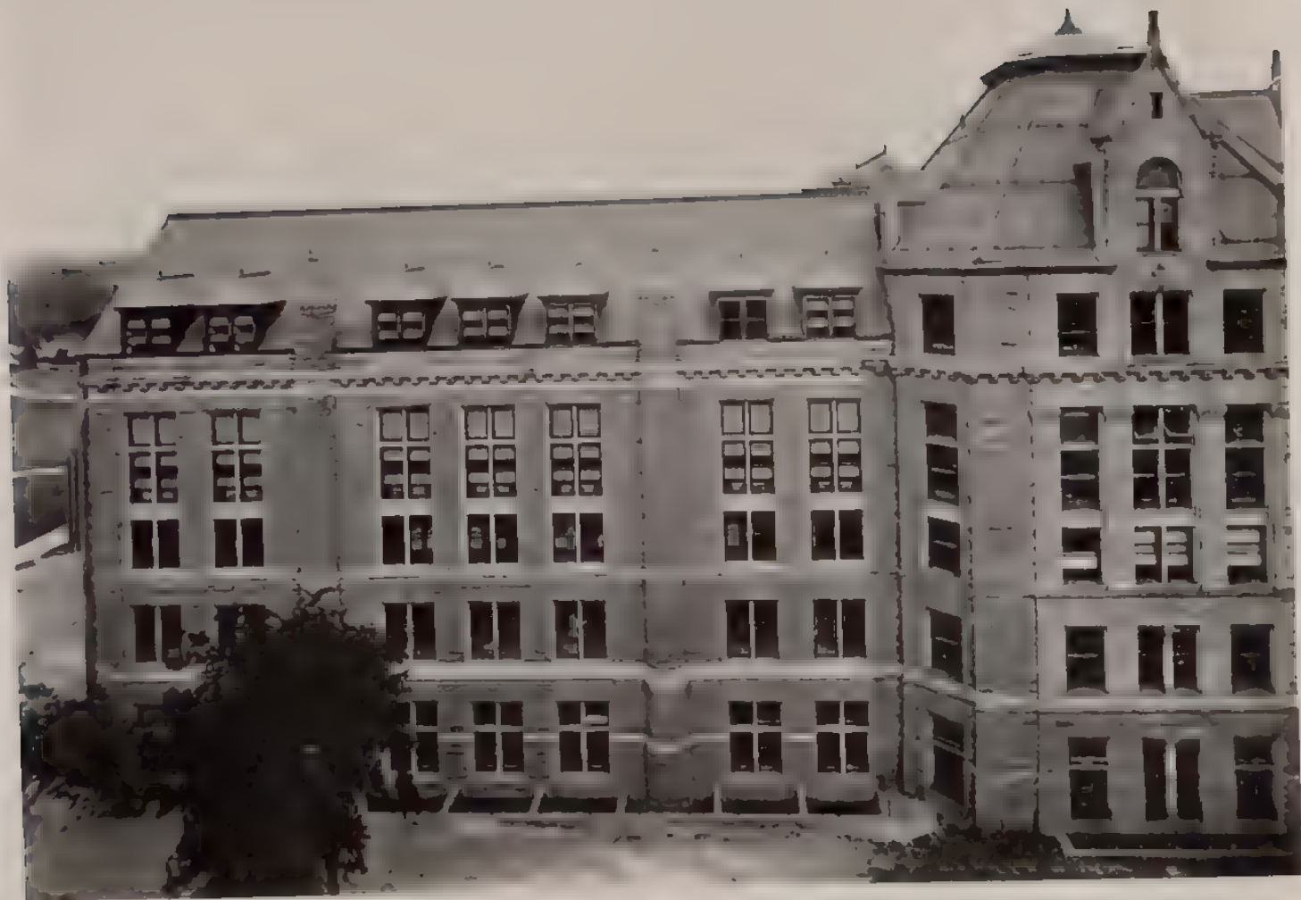
THE MUSEUM. South Wing of West Façade
