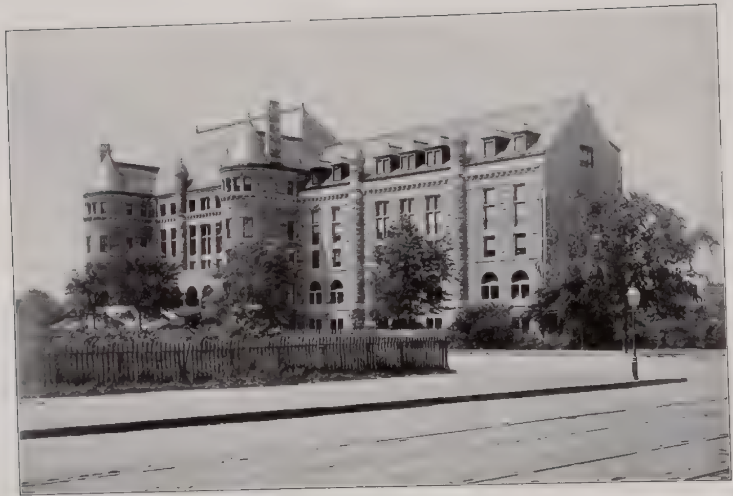
THE MUSEUM. East Wing of South Façade, 1893-1895
