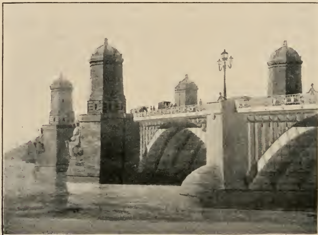
NEW CAMBRIDGE BRIDGE
