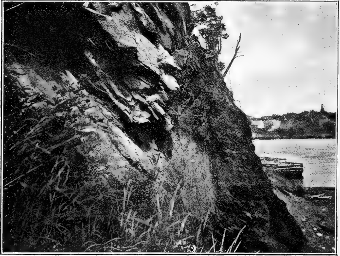
Fault between Tetragraptus shale and Acadian, near Suspension bridge, St. John, N.B.
