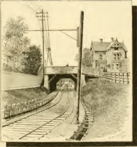
JEFFERSON AVENUE RAILROAD BRIDGE
