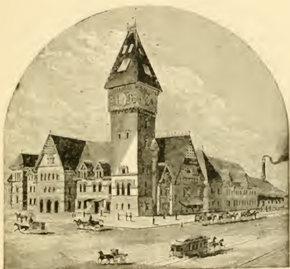
MICHIGAN CENTRAL RAILROAD DEPOT.
