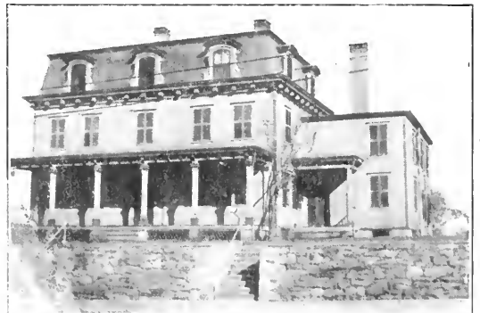
RESIDENCE OF THE LATE WELLS R. RITCH ON ATLANTIC STREET. Built in 1835.
