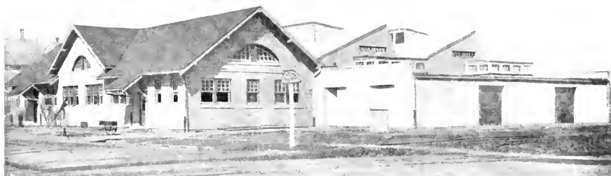
SOME STORAGE AND WORKING BUILDINGS
