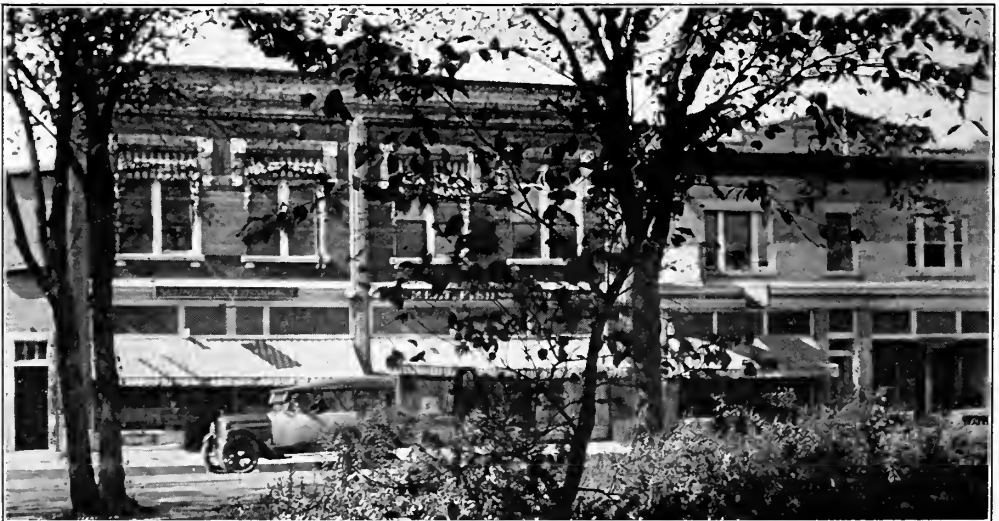
A BEAUTIFUL BLOCK WAS MADE POSSIBLE AND AROSE OUT OF OLD ARCADIA.
