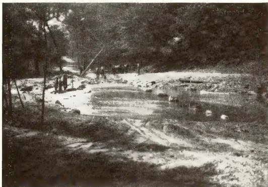
Building the lower ford, view from the east side of the creek, circa 1913.
