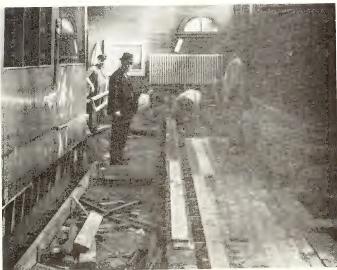
Replacing the floor of the Lion House, completed in 1935.
