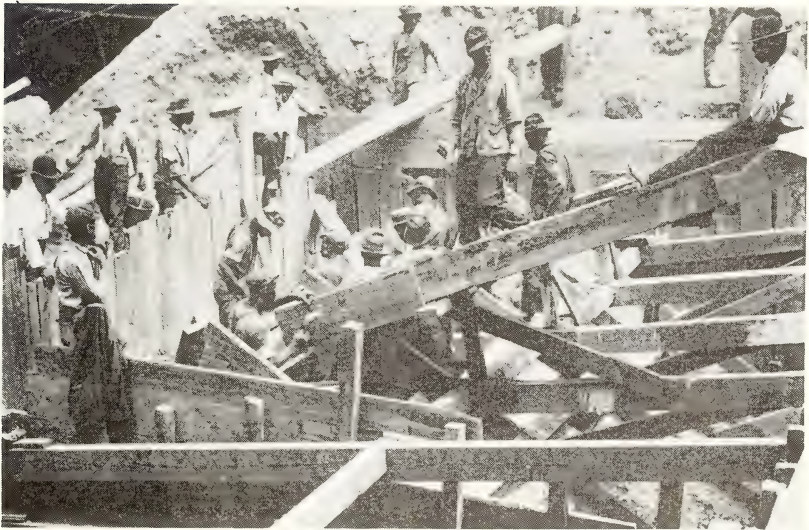
Building a stone bridge, 1913.
