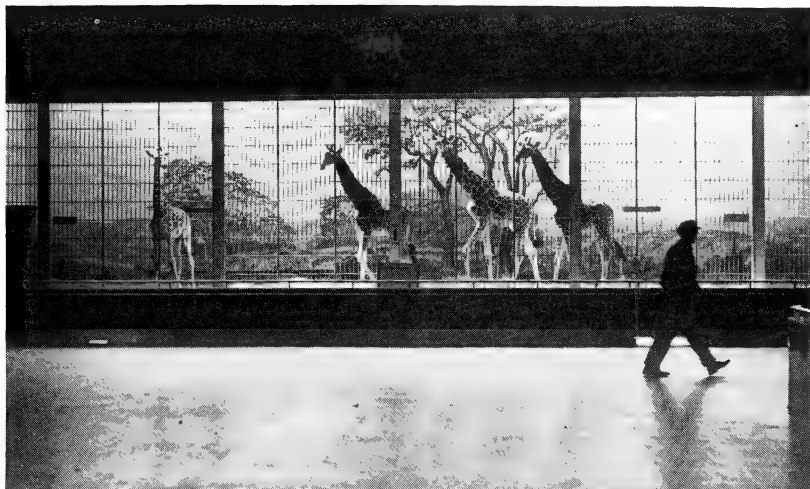
Interior of the Elephant House, constructed during 1936-1937.
