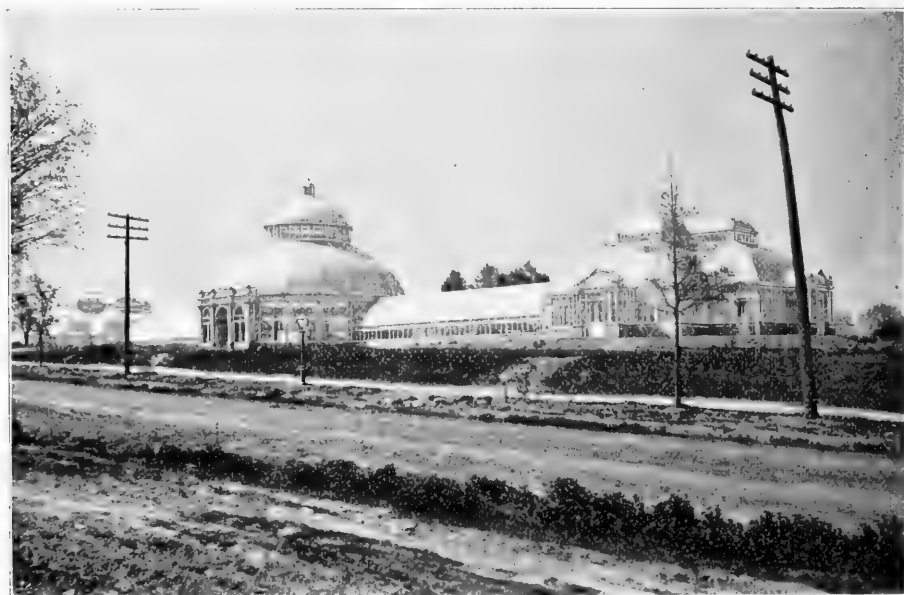
Main Horticultural houses : view from the northwest. New York Botanical Garden.
