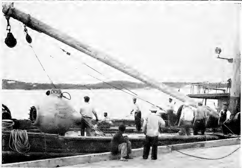
FIG. 61. ( upper ) We are now at the wharf where the bathysphere, winches and miles of cable have lain in their housing for a year and a half. The 3000-foot rubber hose, enclosing the telephone and electric light wires, is just coming aboard. FIG. 62. ( lower ) We see the bathysphere on the deck of the Freedom , and the enormous yard, brought especially from last year's boat. The low bulwarks and wide expanse of deck make this craft ideal for our work. But she proves to be only sea-worthy.
