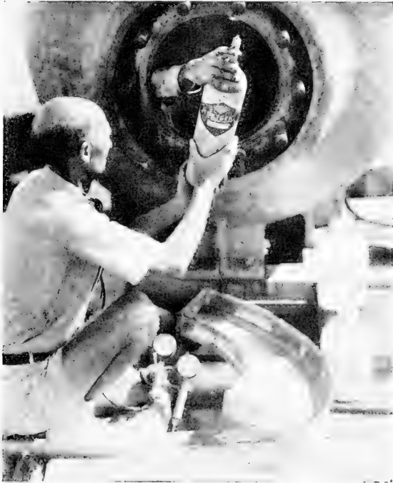
FIG. 76. ( upper ) Another test dive is necessary, and this is made on the morning of September 22nd, a clock being sent down, the ticking audible over the telephone wires. The sphere comes up dry. At the moment of this photograph we are examining every detail of the sphere and watching the unfavorable weather to decide on the possibility of making the broadcasting and our deepest 1932 dive. At 12:55 I decided to risk it. FIG. 77. ( lower ) More rapidly than ever before we begin loading the bathysphere, tightening the stuffing-box, attaching the chemical trays, filling them and installing the oxygen tanks.
